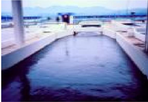
**Figura 2-12.** Canaleta Parshall para  $1,0 \text{ m}^3/\text{s}$  (4)
